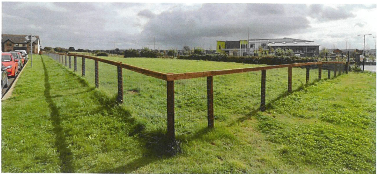
Figure 3: The erected fencing as viewed from the north-west corner.
